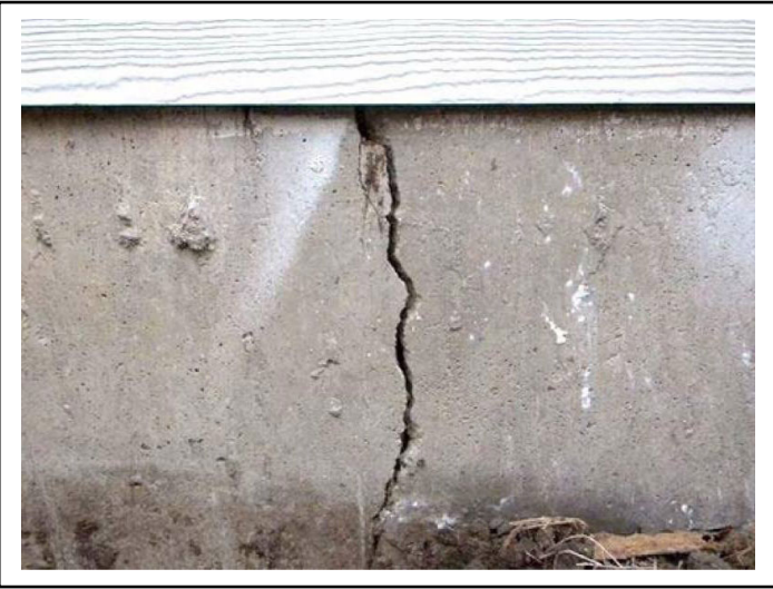
Comment: Observed foundation crack
