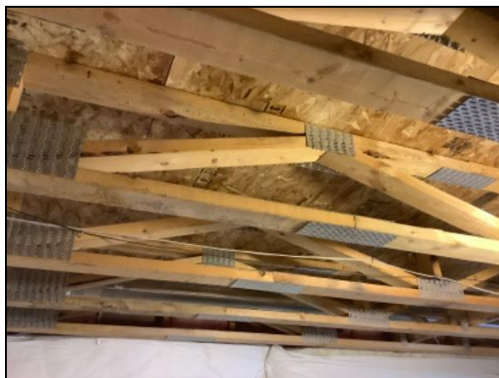
Comment: View of joists in basement
