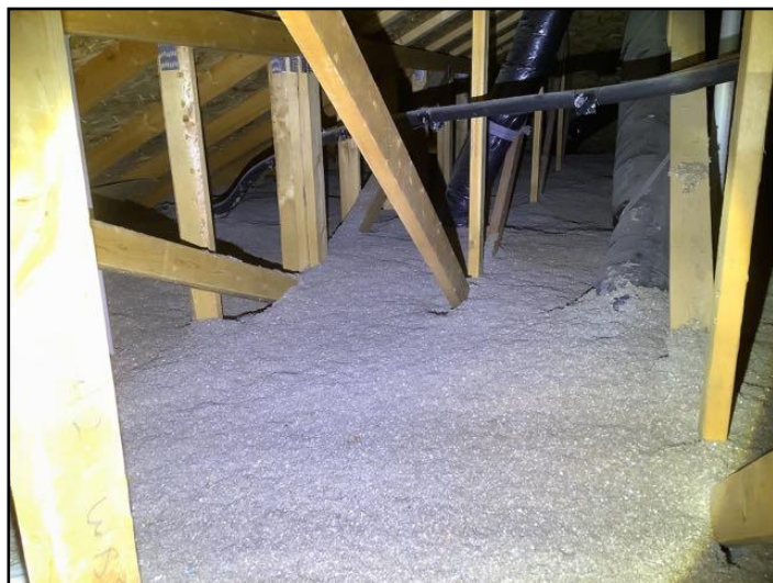
Comment: View of attic structural components
